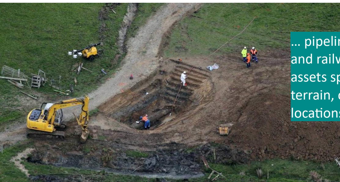
Repairs to the Maui pipeline in Taranaki, 2011 – Cameron Burnell/Stuff
